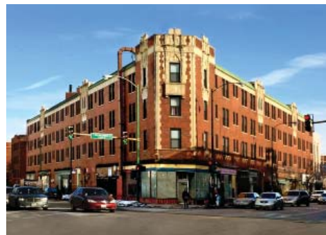
2799 N. Milwaukee – 99 Units Renovated
