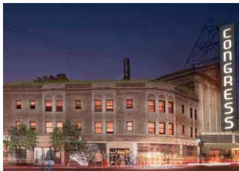
Congress Theater – $55M Renovation
