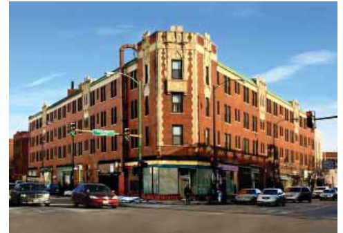
2799 N. Milwaukee – 99 Units Renovated
