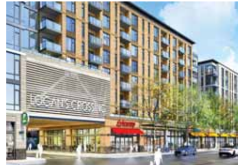
Logan's Crossing – 220 Units Under Construction
