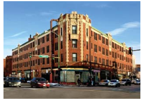
2799 N. Milwaukee – 99 Units Renovated
